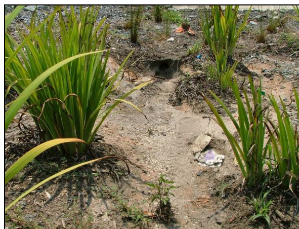
Figure 5-8. Examples of erosion within a Bioretention Basin
