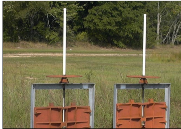
Figure 7-5. Two large sluice gates with PVC covers
