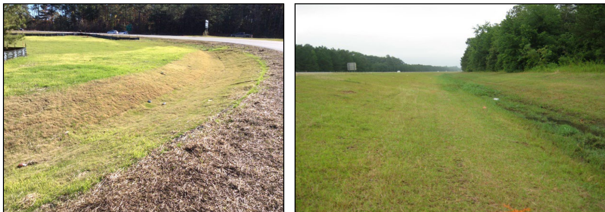
Figure 12-7. Linear highway applications of Swales
