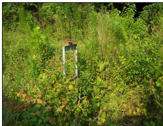
Figure 10-5. A sluice gate barely visible due to overgrown vegetation
