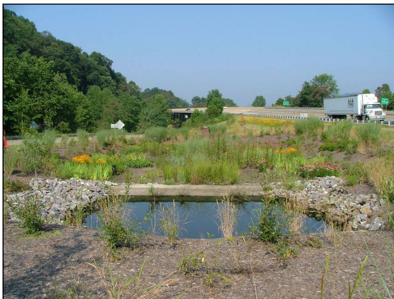
Figure 5-5. Typical forebay (foreground)
