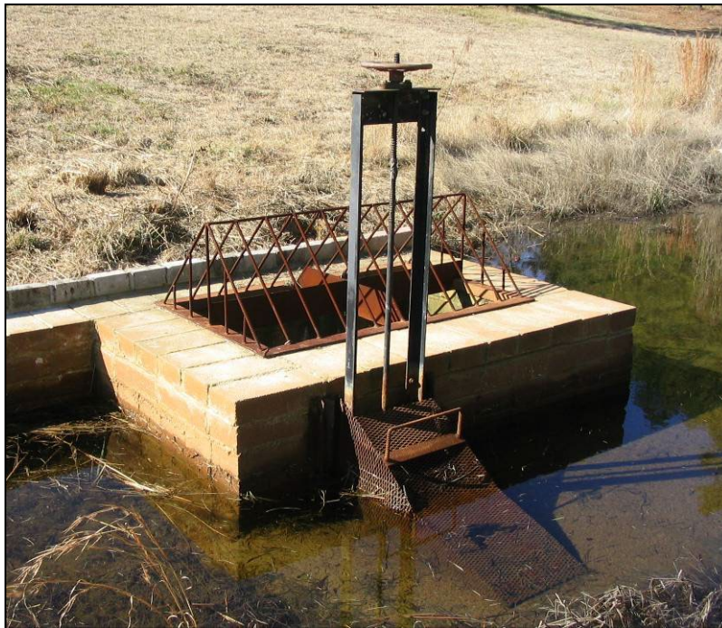
Figure 8-7. An outlet control structure
