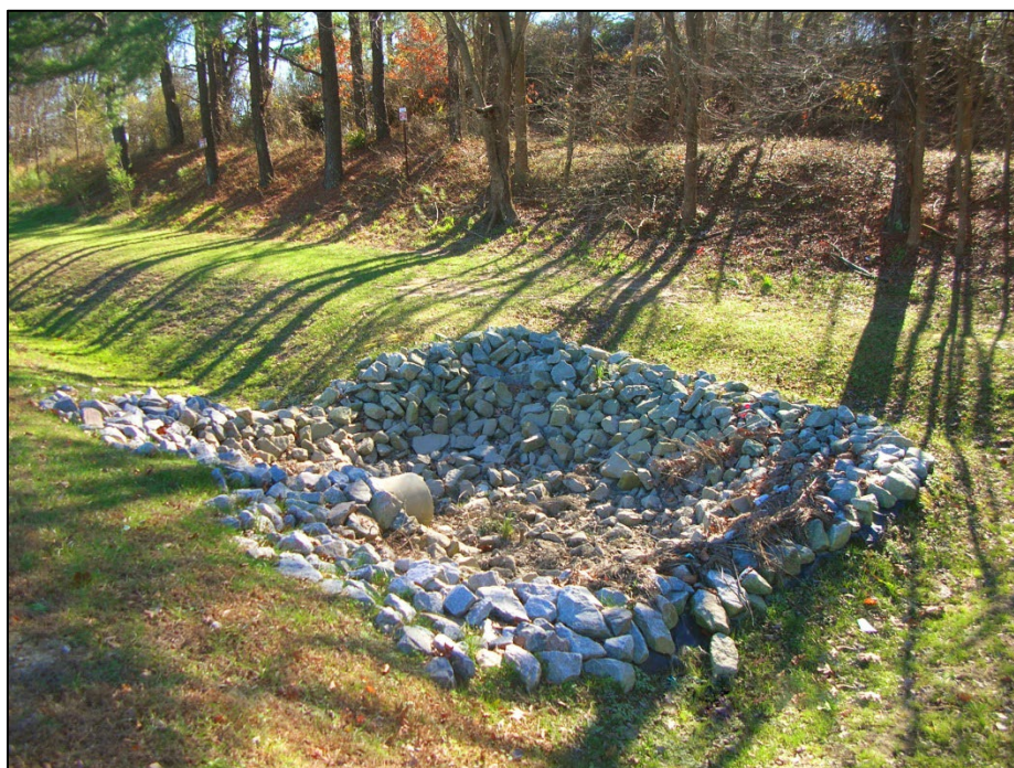
Figure 15-1. Standard Preformed Scour Hole Installation
