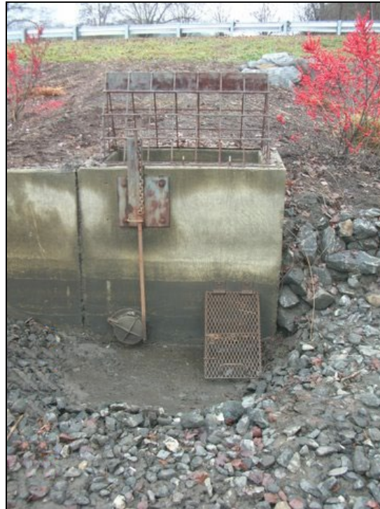
Figure 9-9. A lift-type sluice gate
