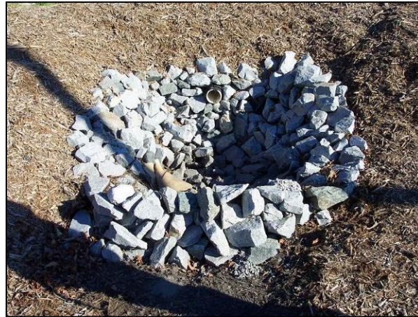
Figure 12-6. A well-maintained forebay
