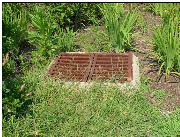
Figure 5-10. Bioretention Basin outlet control structures
