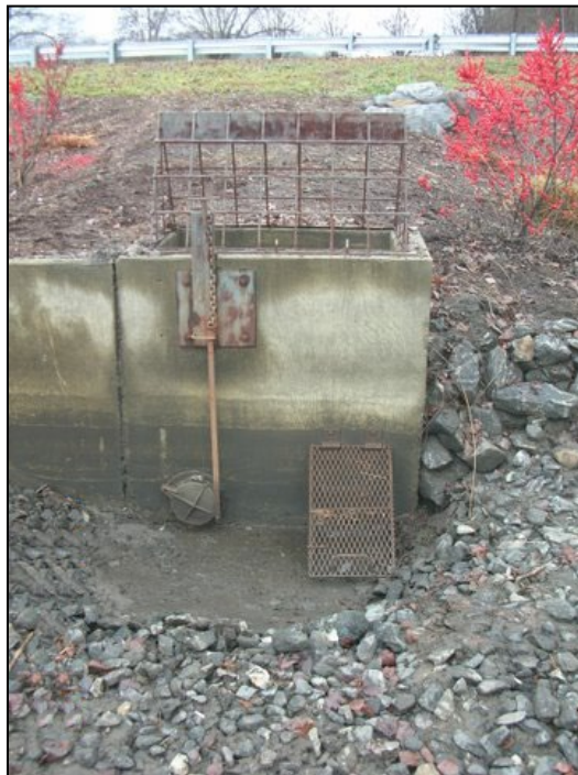
Figure 8-9. A lift-type sluice gate
