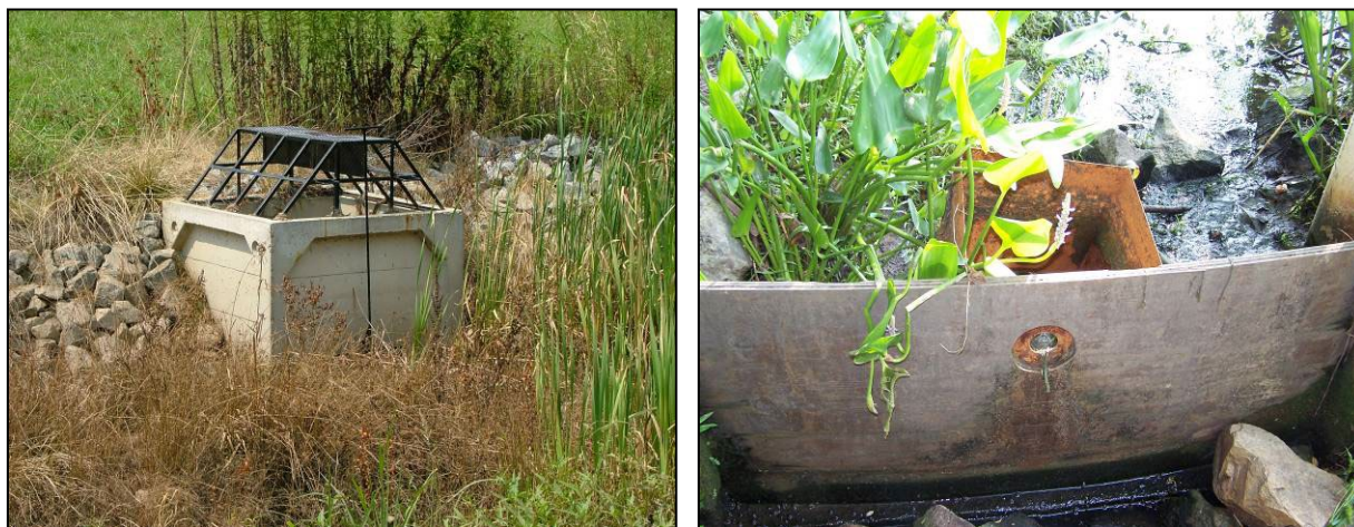
Figure 11-7. Two examples of outlet control structures: a standard riser (left) and a flashboard riser (right)
