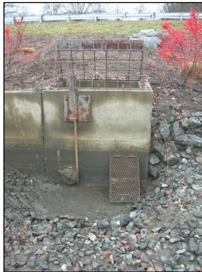
Figure 10-6. Lift-type sluice gate
