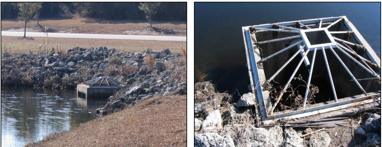
Figure 9-6. Two views of an outlet control structure
