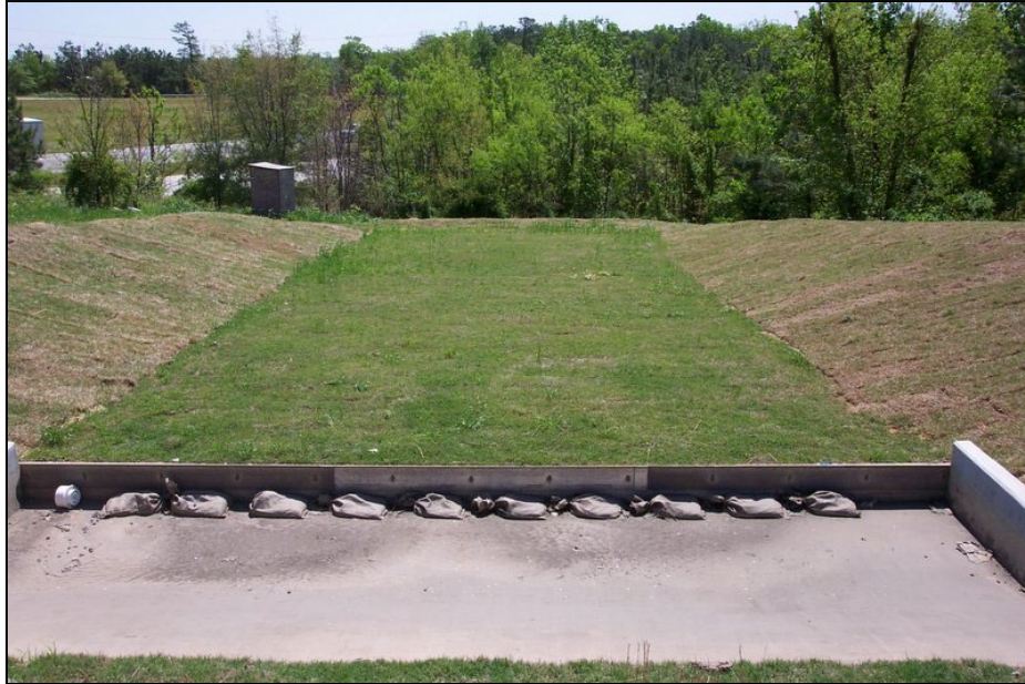
Figure 13-7. Example of a Level Spreader and filter strip with a drawdown device consisting of weep holes with rock bags
