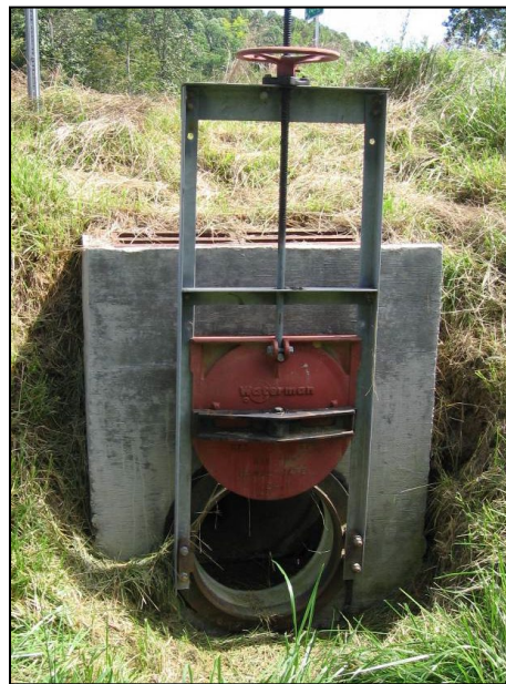
Figure 9-8. An open screw-type sluice gate
