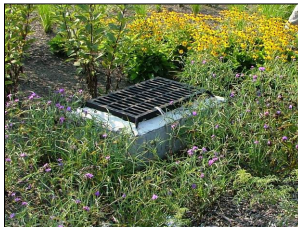
Figure 5-10. Bioretention Basin outlet control structures
