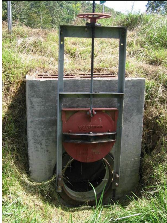
Figure 11-8. An open screw-type sluice gate
