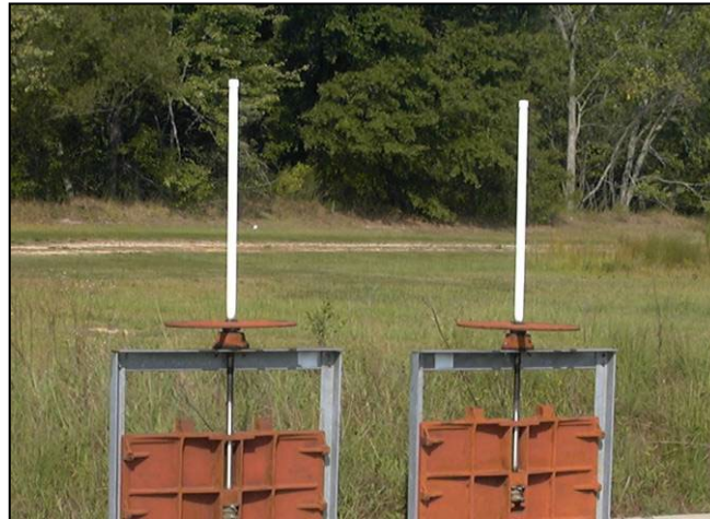
Figure 11-10. Two large sluice gates with PVC covers
