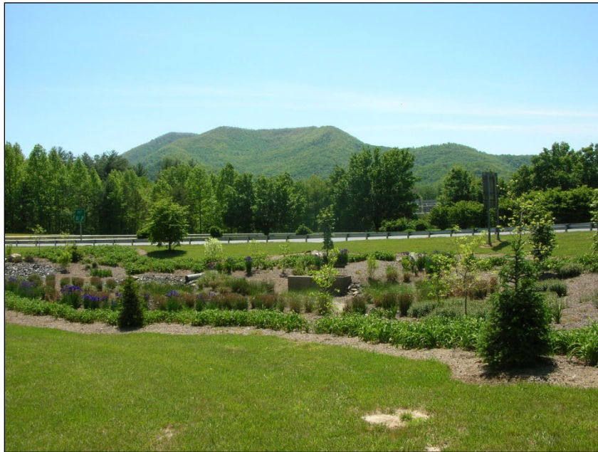
Figure 8-5. Dry Detention Basin with planted landscaped vegetation
