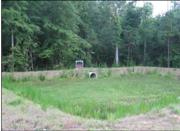
Figure 10-8. A sluice gate mounted on the downstream end of the outlet pipe
