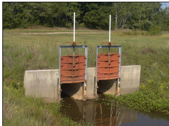
Figure 10-7. Large, screw-type sluice gates with PVC cover and cap over worm gear
