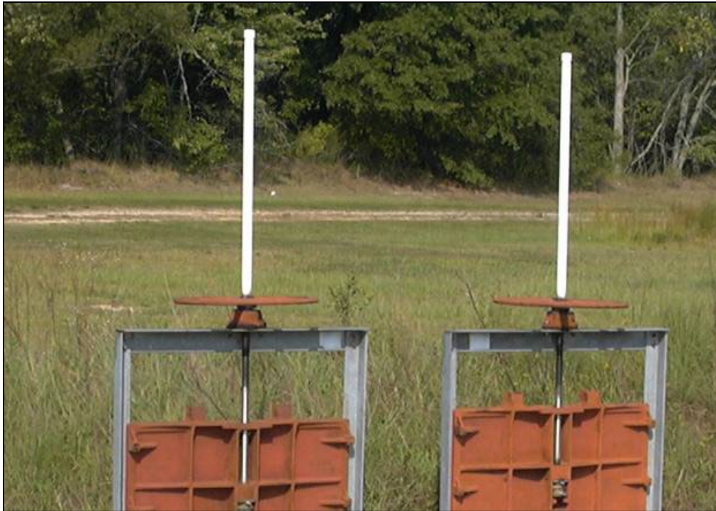
Figure 6-6. Two large sluice gates with PVC covers
