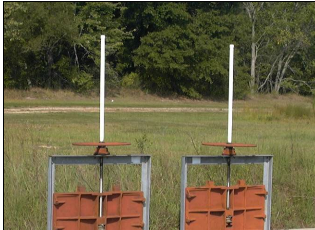
Figure 9-10. Two large sluice gates with PVC covers
