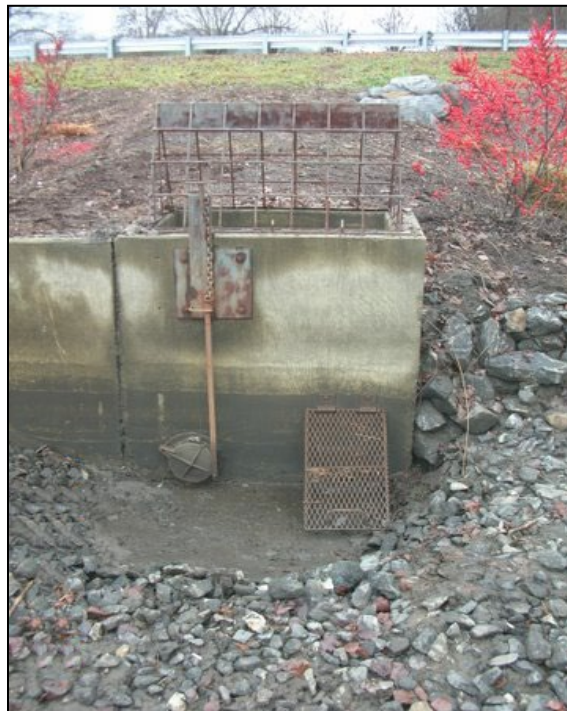
Figure 11-9. A lift-type sluice gate
