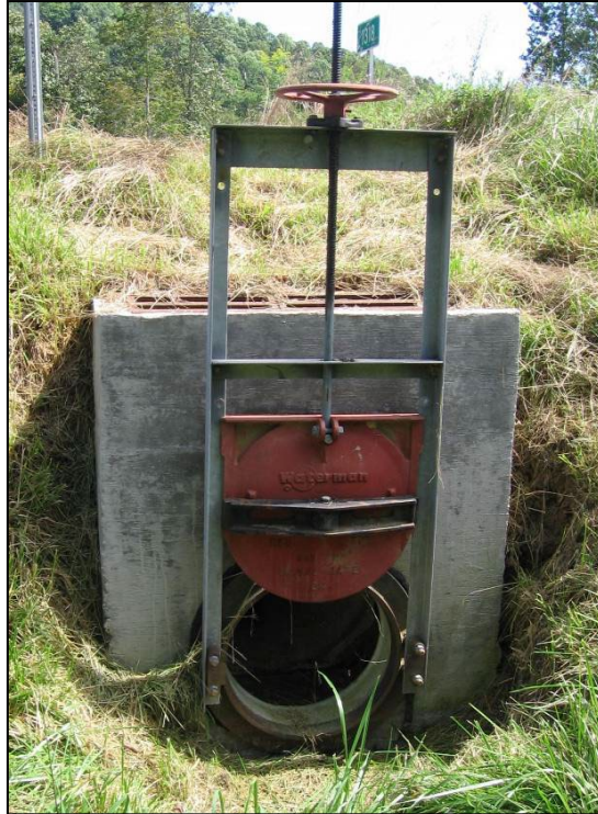
Figure 8-8. An open screw-type sluice gate
