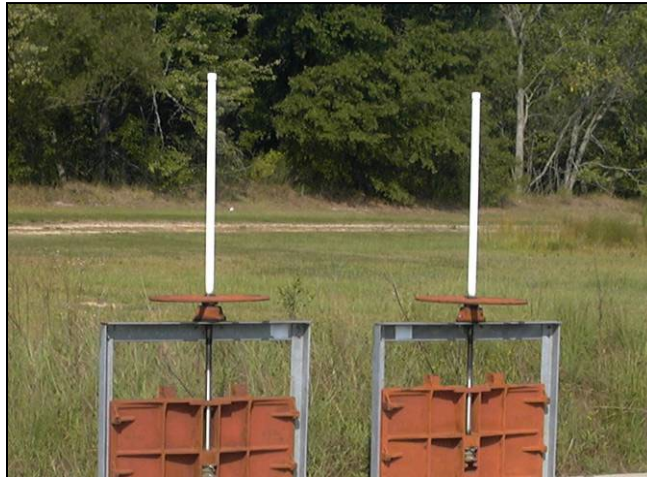
Figure 8-10. Two large sluice gates with PVC covers
