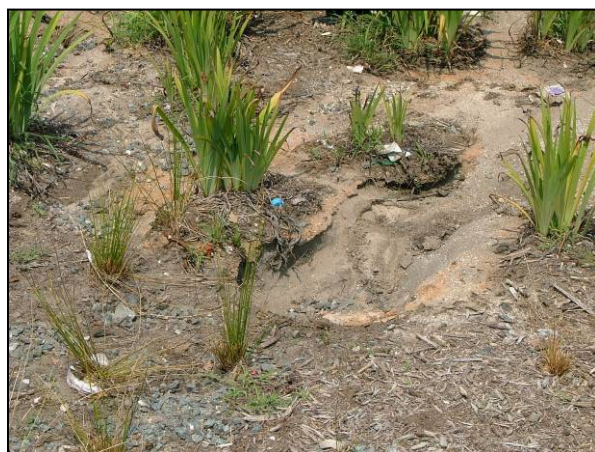
Figure 5-8. Examples of erosion within a Bioretention Basin
