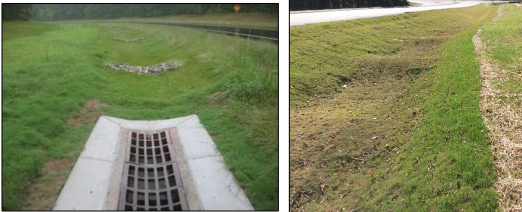
Figure 12-8. Swale with check dams (left) and Swale with false sumps (right)
