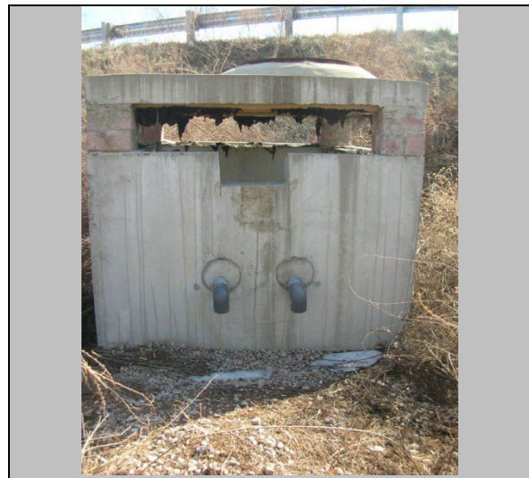
Figure 9-7. Outlet control structures showing two types of drawdown devices, slotted (left) and PVC elbow (right)
