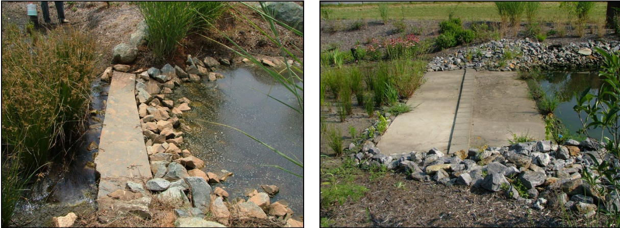
Figure 5-6. Two examples of transition weirs
