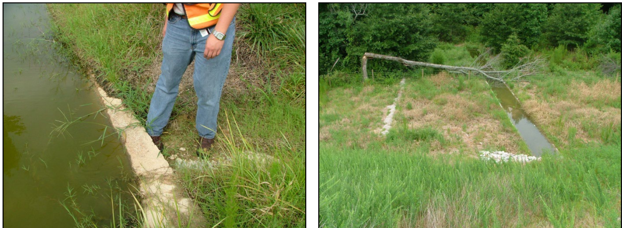
Figure 13-6. Typical maintenance concerns: erosion at the Level Spreader lip and channelization in the filter strip (top), and woody debris in need of removal (bottom)
